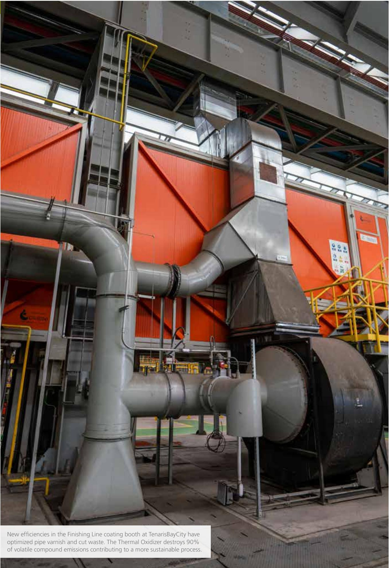
New efficiencies in the Finishing Line coating booth at TenarisBayCity have optimized pipe varnish and cut waste. The Thermal Oxidizer destroys 90% of volatile compound emissions contributing to a more sustainable process.
